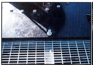
Item No. 14: Replace missing nut on base plate Pump No.2.
